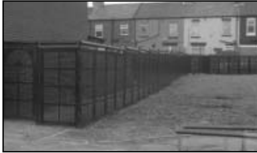
Alley gates, installed extensively in Liverpool, England, have proven a cost-effective method of reducing residential burglaries.
